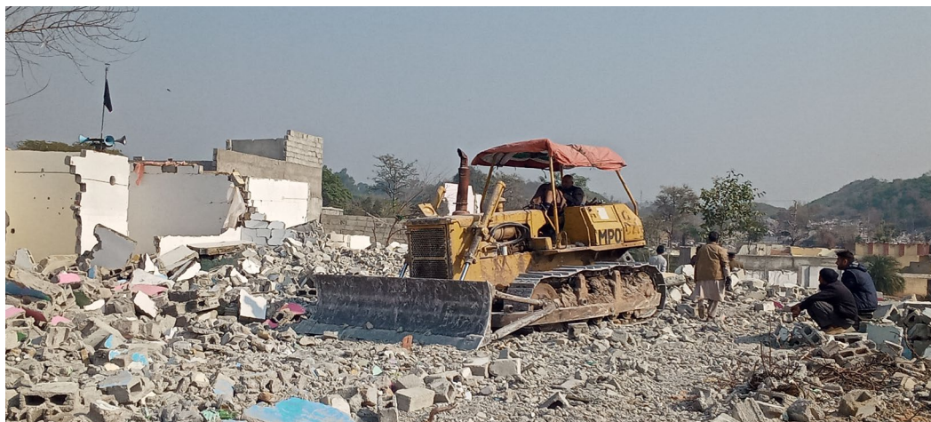
Figure 1. CDA bulldozer demolishing informal houses
