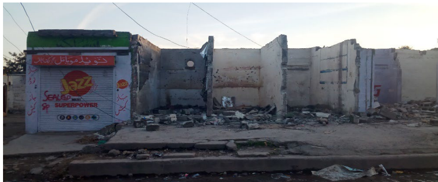
Figure 3. Demolition view of shops operated by small-scale economic operators
